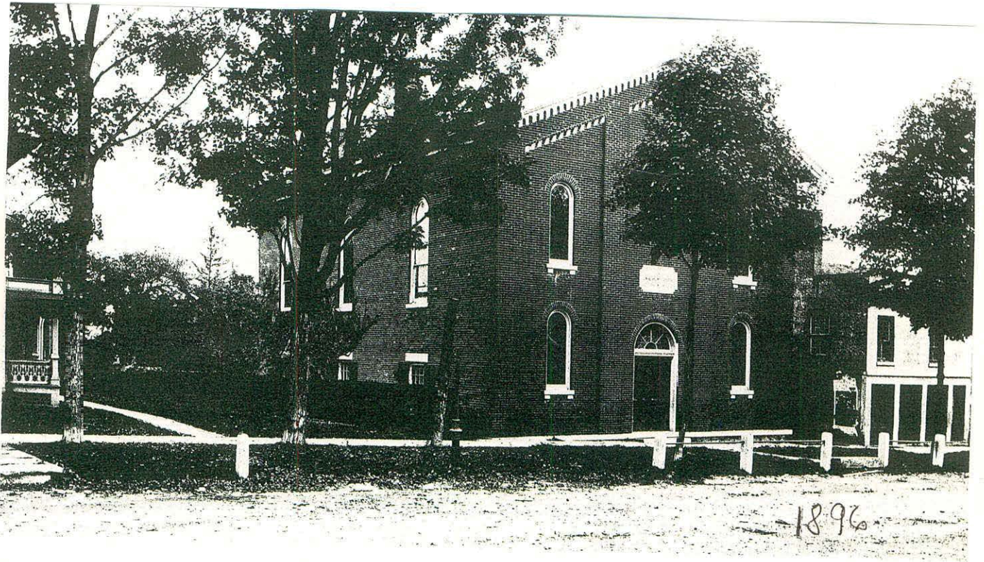
UNIVERSALIST CHURCH LEROY, GENESEE COUNTY, NY
